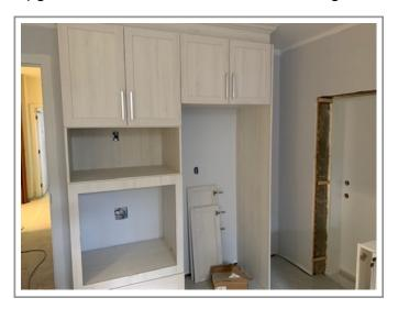
The new door opens into the store room instead of the kitchen. In the next few weeks the counter and backsplash should be installed. Under the new window in the kitchen there will be three full size sinks for proper washing.
